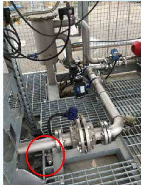
Ektimo used the sampling points shown to collect samples directly into a canister which reduced contamination or air exposure.
