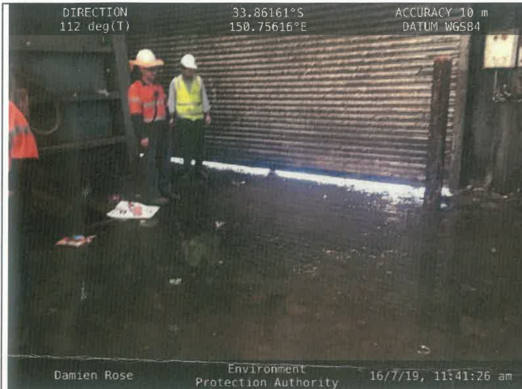
2. Leachate pooling against the roller door
