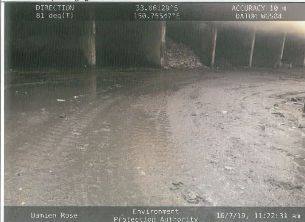
3. Leachate discharging from tunnels without doors
