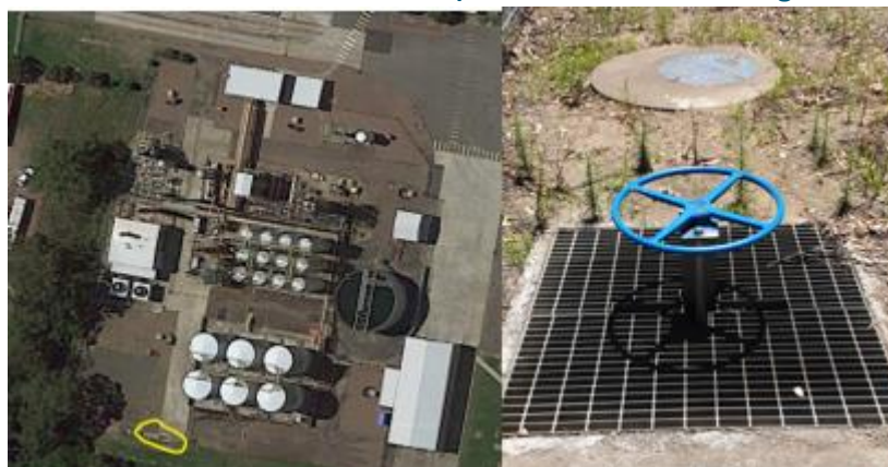
Figure D2: Stormwater Shut off valve (from Stormwater Management Plan)
