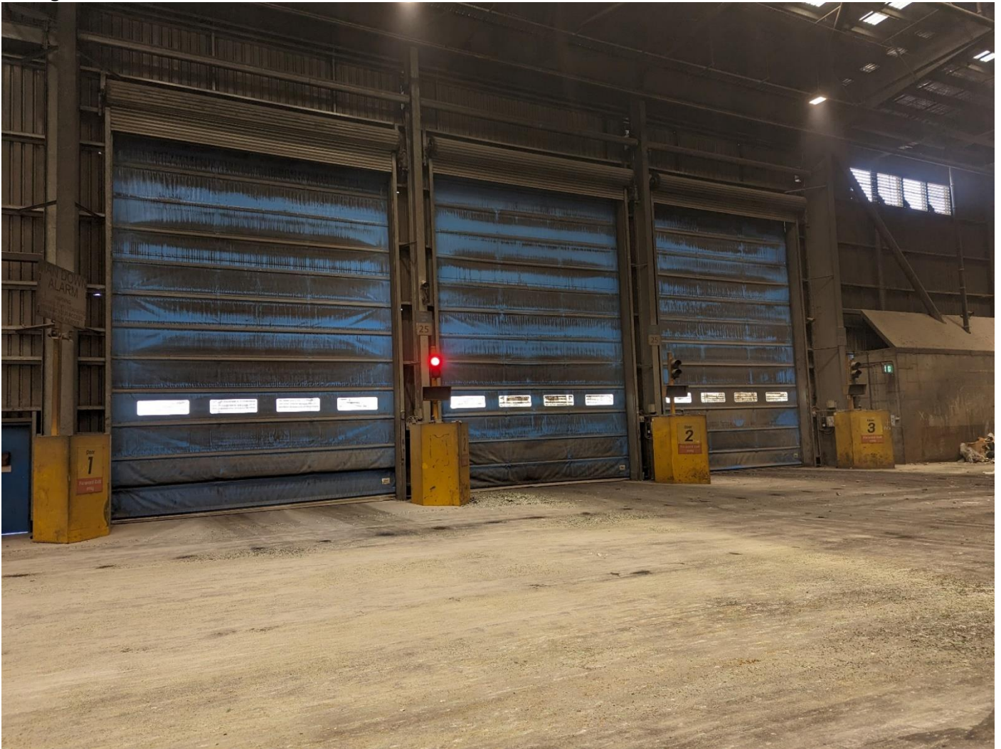
Figure E3. Photograph showing the three rapid roller doors which are kept closed unless trucks are entering or exiting the WTS.
