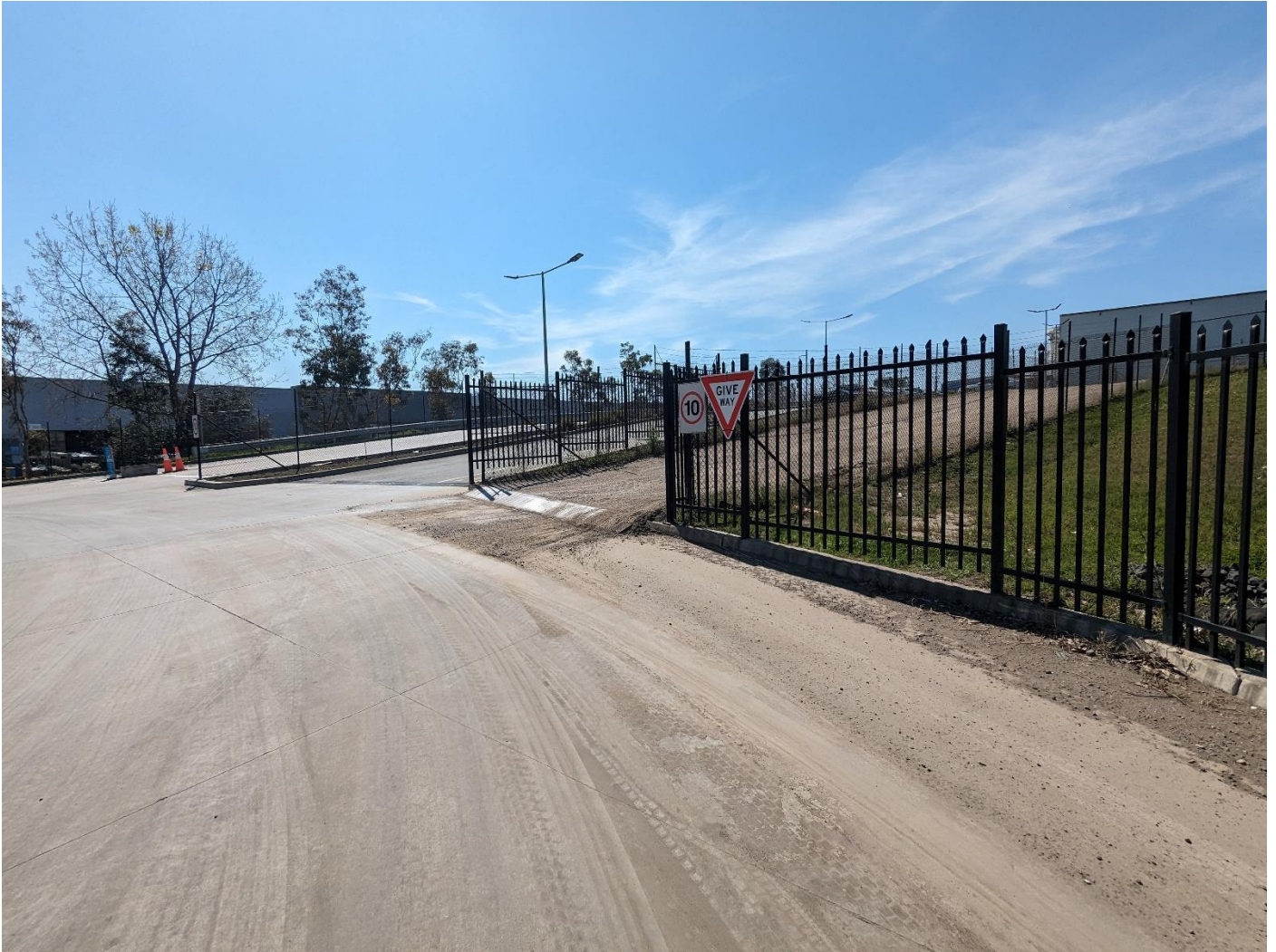
Figure E4. Photograph showing the unsealed access road to the Stage 2 area which is causing sediment to accumulate at the front of the Site.
