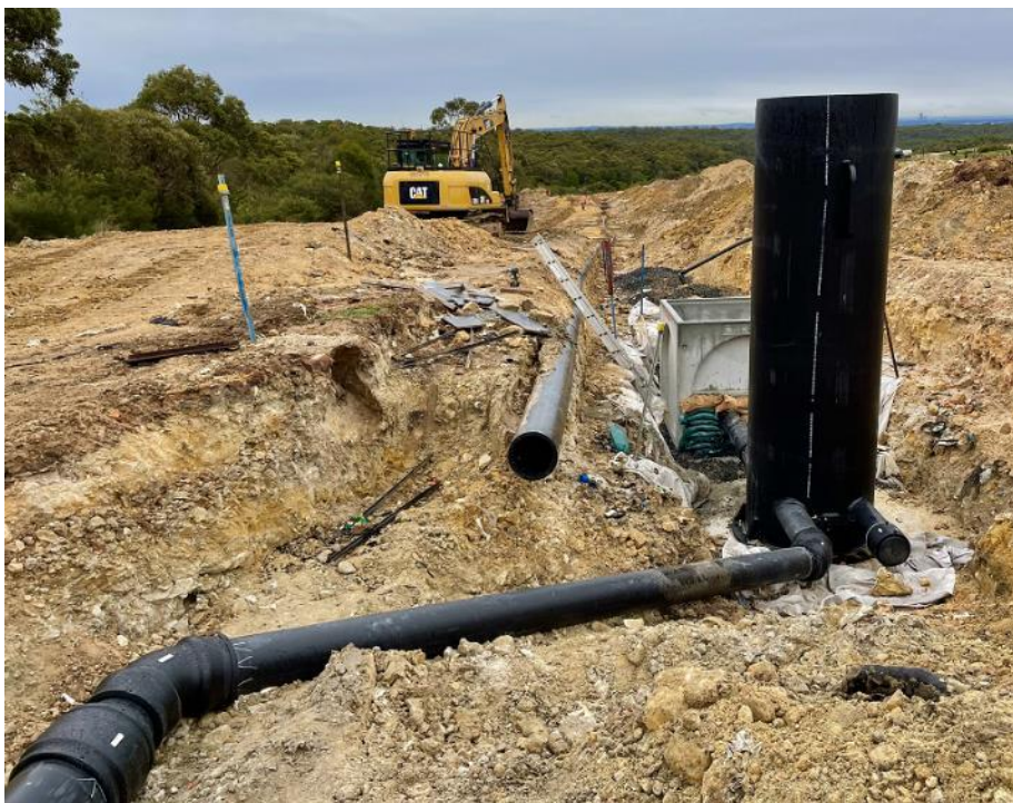
Leachate/Gas cut-off trench installation at Area G
