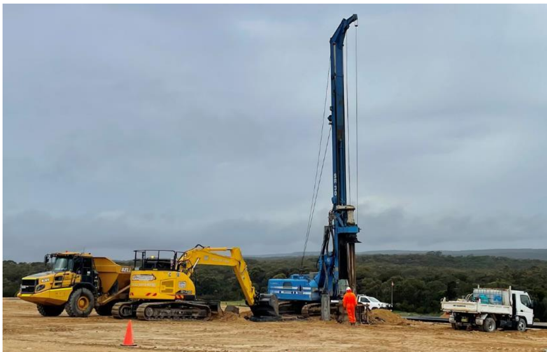
Gas well installation in Area A
