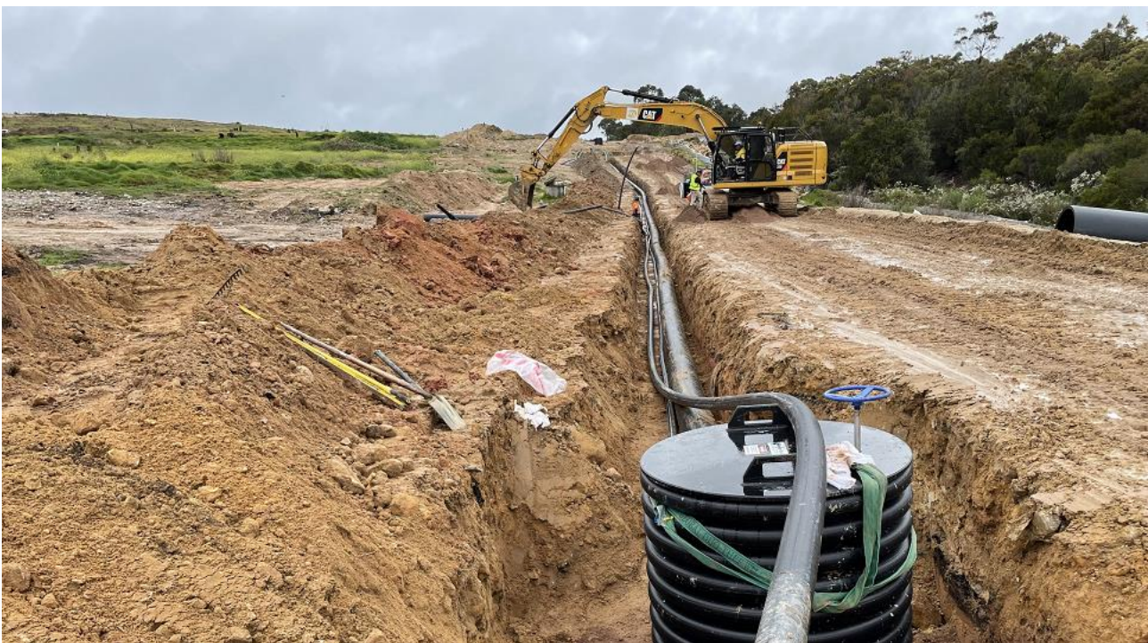
Gas header pipe installation in area G
