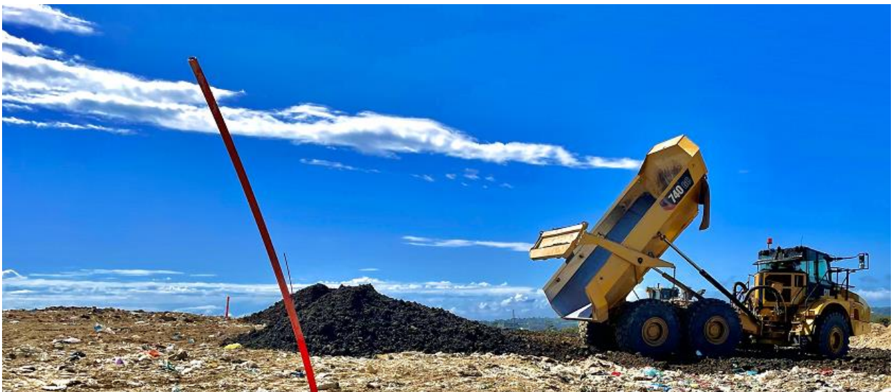
Installation of Seal Bearing Layer at Area A
