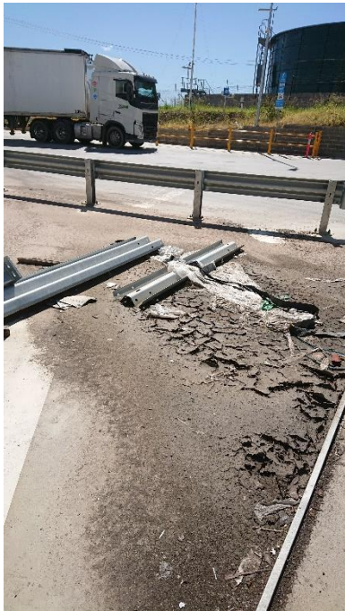
Figure F1.2. Evidence of litter / sediment accumulation in front of Waste Transfer Station (eastern side) (left) and along the batter associated with the south east corner of the site (middle). Some evidence of soil tracking onto hardstand areas along southern exit of site (right). Site inspection 06/04/20.
