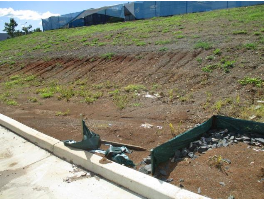
Figure F1.7. Soil erosion occurring in landscaped areas along southern and western side of site, with some little accumulation on stormwater pits. Site inspection 06/04/20.
