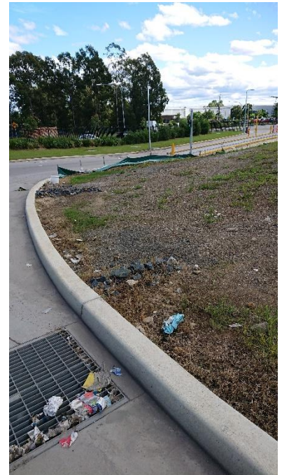
Figure F1.7. Soil erosion occurring in landscaped areas along southern and western side of site, with some little accumulation on stormwater pits. Site inspection 06/04/20.
