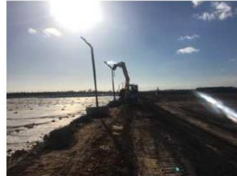
Litter fence being installed at MRL
