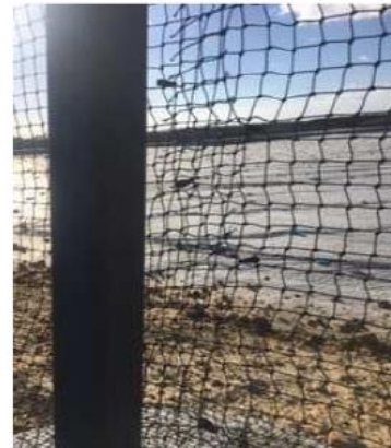
Netting overlapped and clipped at each post
