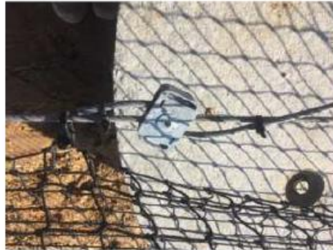
Gripper to tension the 6mm wire core cable – can be re-tensioned or released to relocate the nets
