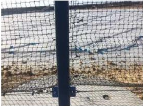
Netting overlapped and clipped at each post
