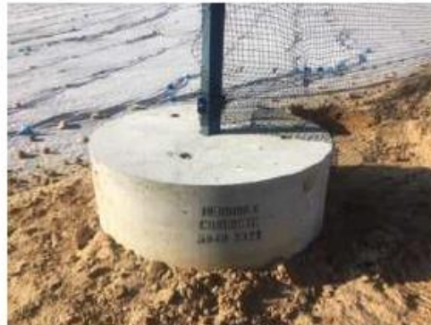
Posts slip into concrete base sleeves – Bases 1.5 in diameter and weight 2.5 ton
