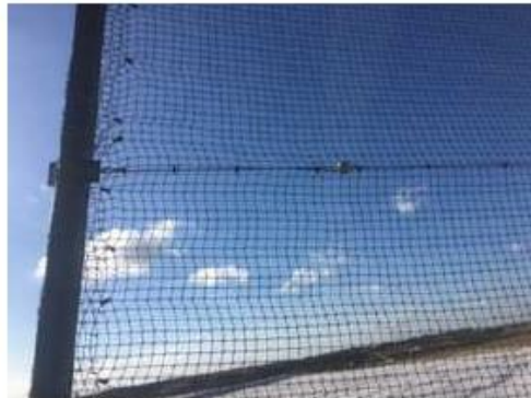
Clipped net with 6mm wire cables and tensioned using gripples.
