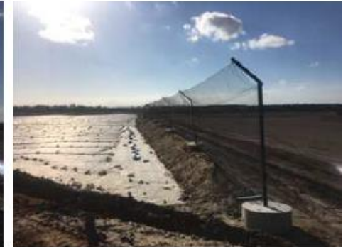
New litter nets being installed at MRL
